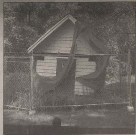
An old smokehouse which is being restored.
