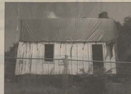
A log cabin from the early 1800s is covered by siding to protect the wood. It will be moved to a new wooded plot.
